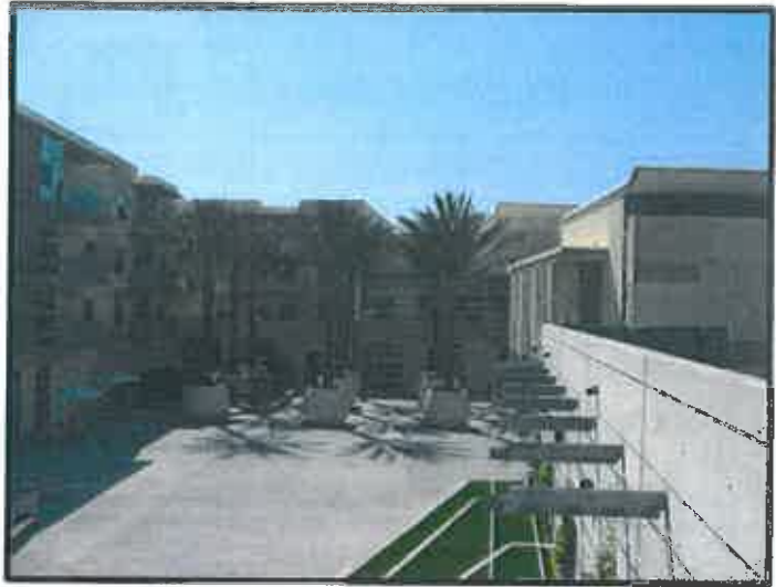
Figure 2: Courtyard Overlying Podium Parking Structure
